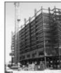
Marriott Hartford Hotel under erection. Photo by Corley
